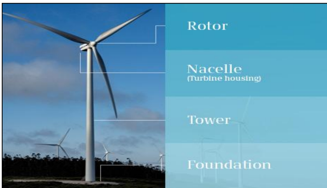
Plate 2-1 Wind Turbine Components
