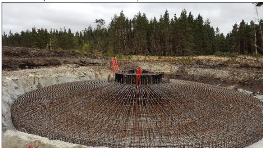
Plate 2-2 Turbine Foundation Anchor Cage surrounded by reinforcing steel.
