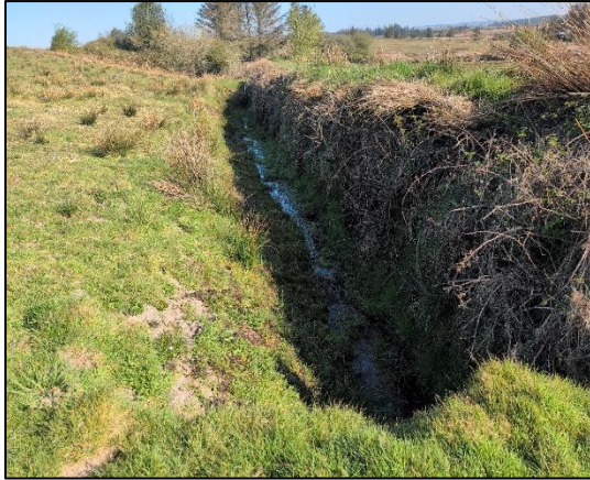
Plate 3-28 Drainage ditch (FW4) on a field boundary
