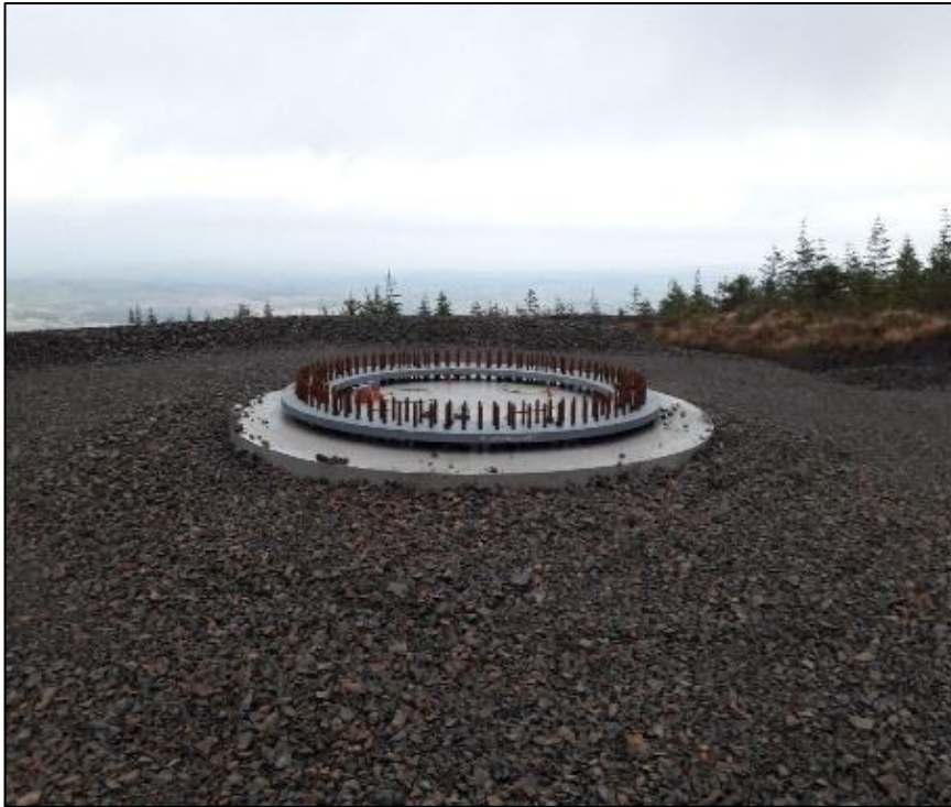
Plate 23 Finished Turbine Foundation
