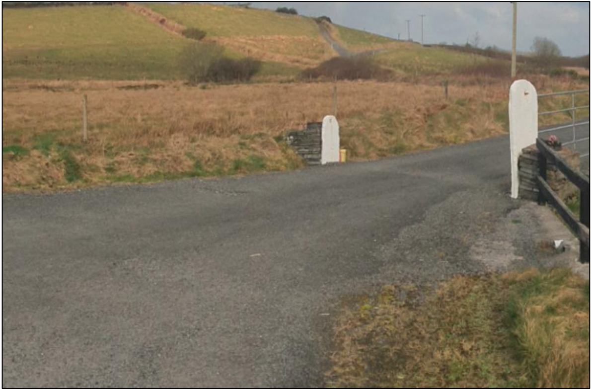
Plate 3-42 Location of accommodation works to the north of Site, showing rush dominated Wet grassland (GS4).
